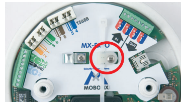
Prepare the cable ties
